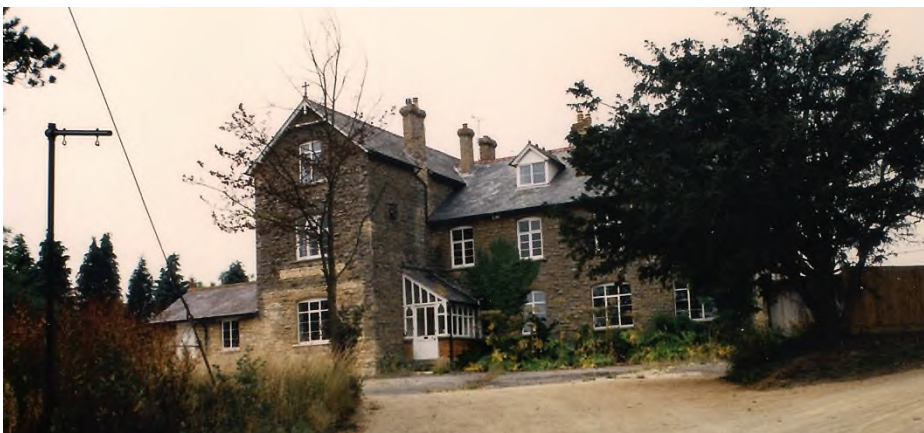
St Michael's shortly before demolition in 1989
