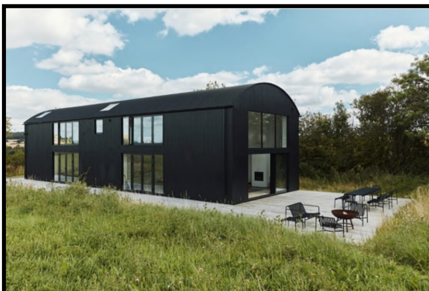
Figure 11: Converted Dutch Barn at Long Compton, photo courtesy of The Modern House ( www.themodernhouse.com ).
