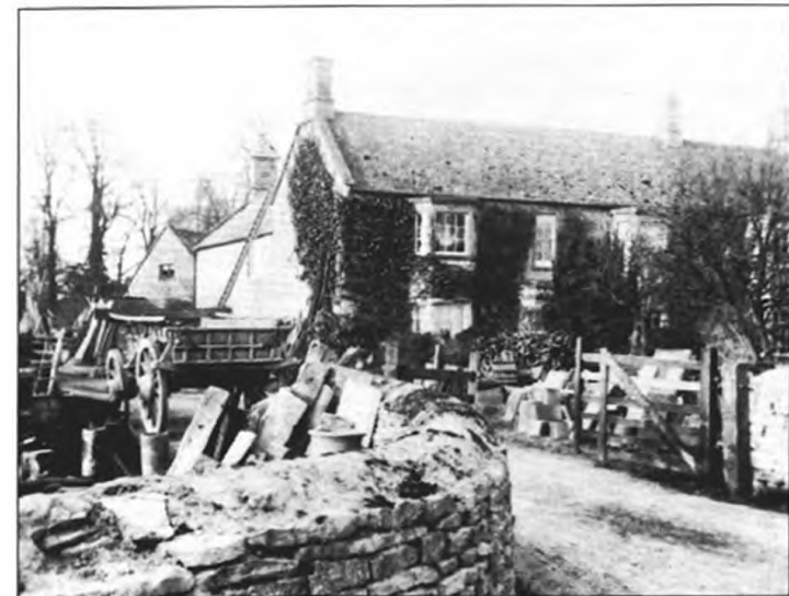
The Elms, Milton under Wychwood, a farmhouse and also the site of Groves' masonry business
