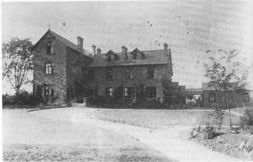
St Michaels, Milton Road, Shipton, has seen more changes than most. This late Victorian building was used as a College for Young Ladies in the last century and then as a home for waifs and strays. Since the 1930s it has been used by Basque refugees, the army and was the proposed site for the Wychwood Social Centre. It then became a corn chandlers, a warehouse and mill, an antique shop, a guest house and now faces an uncertain future
