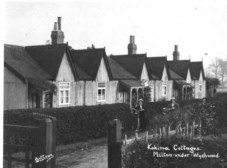
Kohima Cottages, Lyneham Road, Milton, probably 1920s. The cottages were built in 1893 by the widow of Colonel Damant who was killed at Kohima in 1857 during the Indian Mutiny. Mrs Damant wanted to help other widows of the mutiny during their last years and built the row of six one-bedroomed cottages on land adjoining her house, now Heath House. Corrugated iron, a revolutionary building material at that time, was used for both the outer walls and the roofs. It is likely that the cottages were one of its first applications. Flush toilets and mains water were added in 1929.
