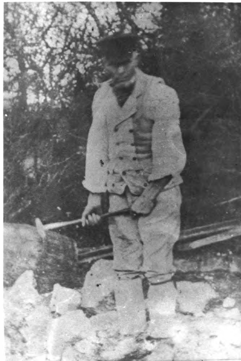
Ben Pratley stone breaking, about 1900. Ben Pratley was a Milton quarryman who lived in Magpie Alley off Church Street, Shipton. He was a quarry mason which ranked between a building mason and a field mason.
