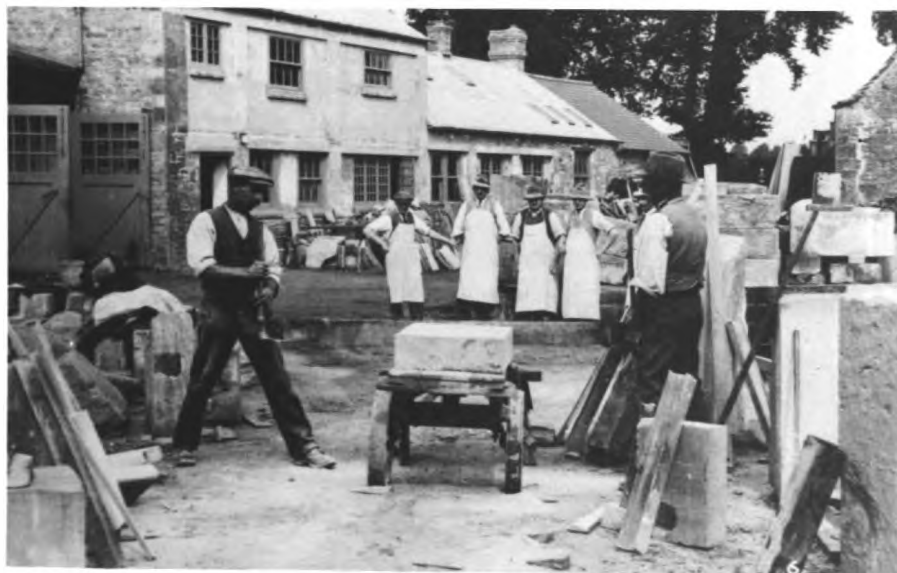
Stonecutters at Groves' Yard, 1926. Jim Puddle and Ned Rathband are using a cross-cut saw to shape the stone. Stonemasons Bill Yateman, Thomas Groves, Alfred Sheppard and Leslie Townsend stand in the background.
