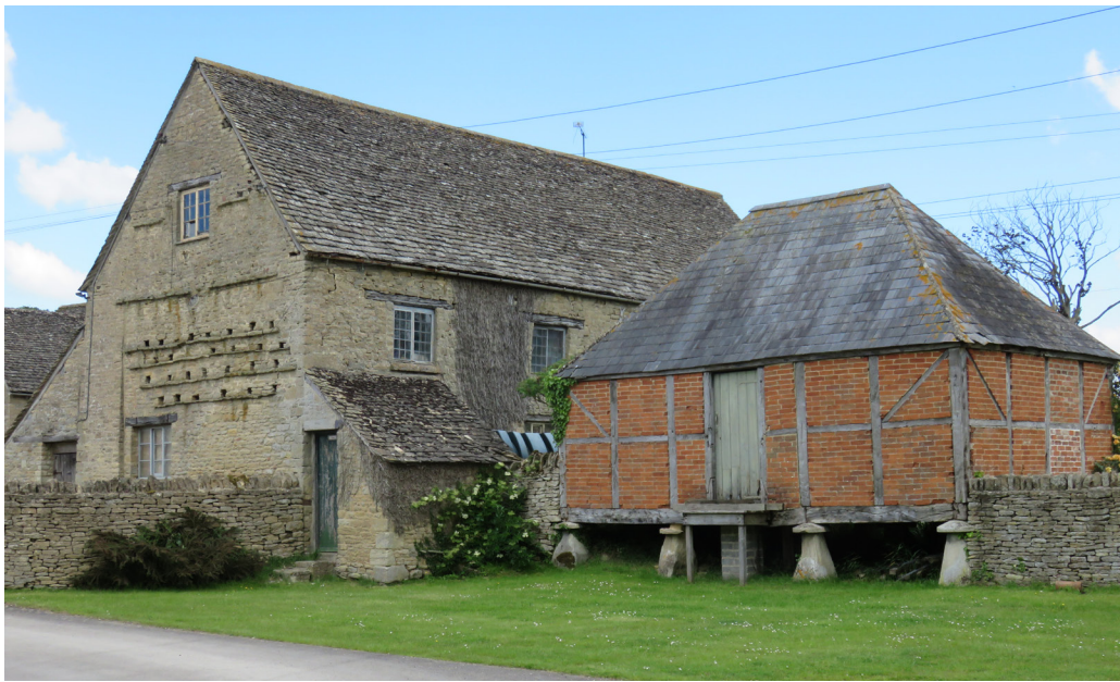
Manor Farm dovecote and granary
