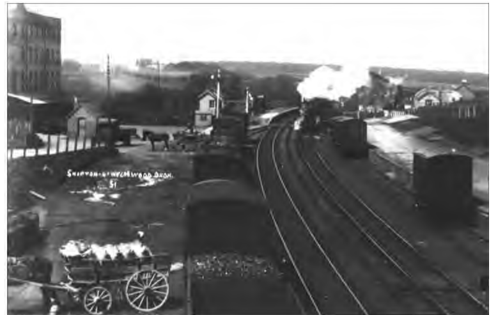
SHIPTON STATION C1920-5. A PASSENGER TRAIN IS PASSING THE UP PLATFORM. THE DOWN GOODS SIDING IN THE CENTRE TOOK UP TO 22 TRUCKS. THE SINGLE TRUCK ON RIGHT-HAND SIDE OF PICTURE WAS FOR HORSES BROUGHT BY HUNTING PASSENGERS.
