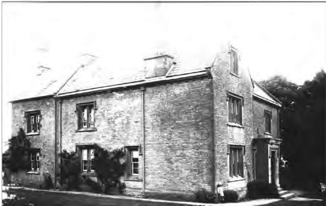
HIGH LODGE, MILTON UNDER WYCHWOOD, ABOUT 1910-15. BUILT AFTER THE ENCLOSURE OF THE MILTON OPEN FIELDS IN ABOUT 1860 FOR ONE OF SQUIRE
