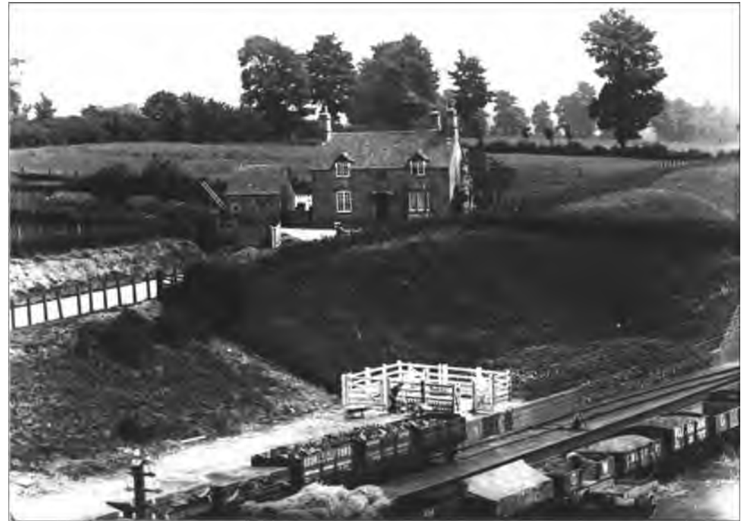
PIKE HOUSE BY THE ROAD BRIDGE WAS ONCE THE TOLL HOUSE FOR THE TURNPIKE ROAD – NOW THE A361. IAN MATTHEWS LIVED AT OAK LODGE FURTHER UP THE HILL, THE GARDEN OF WHICH (BY THE 1930S) RAN BEHIND PIKE HOUSE AND RIGHT UP TO THE RAILWAY LINE. THE STOCK PENS ARE NEXT TO THE GOODS SIDING.
