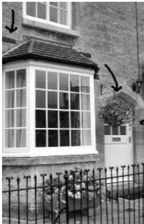
THE OLD WOODEN LINTELS VISIBLE ABOVE THE GEORGIAN BAY WINDOW.
