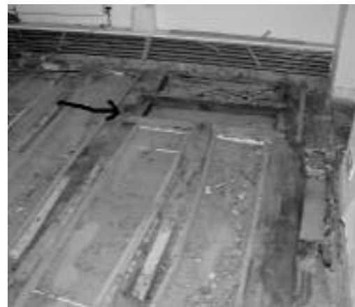
POSITION OF A FORMER STAIRCASE AS SEEN FROM THE ROOM ABOVE.
